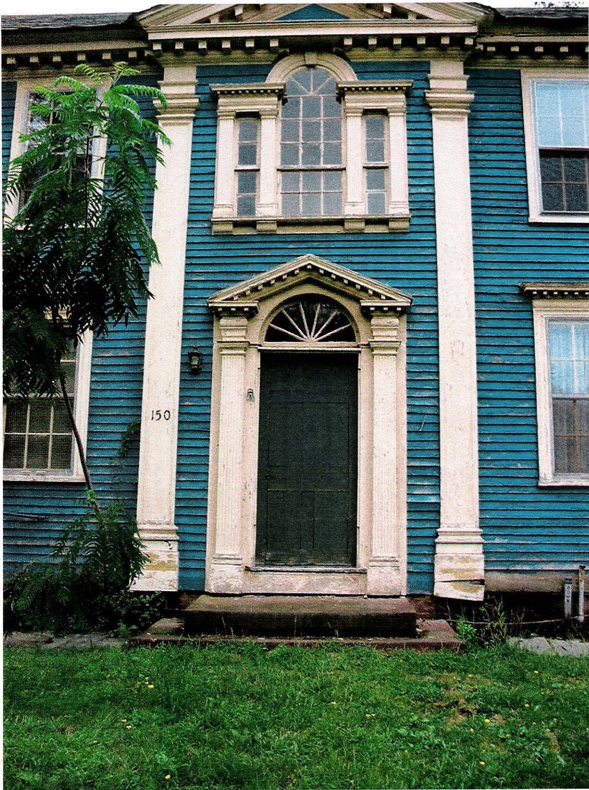
Peters House - 150 East Street – front façade
